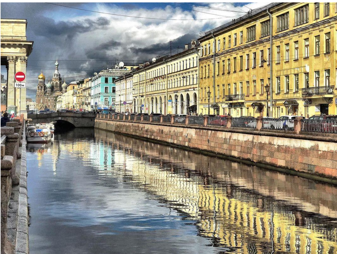
Figure 16. Mistakes in reconstruction of river lining in historical centre of St Petersburg 2021.
